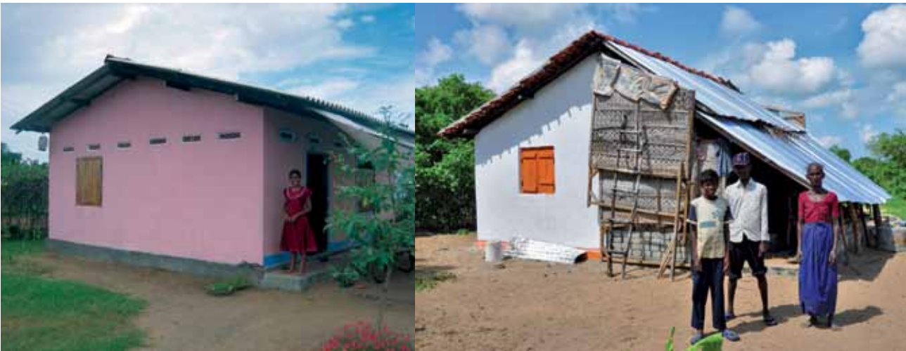
Above - the revised core shelter designs were also upgraded by their new owners. Photos: Varatharajah Ramesh and Glenn Costes
