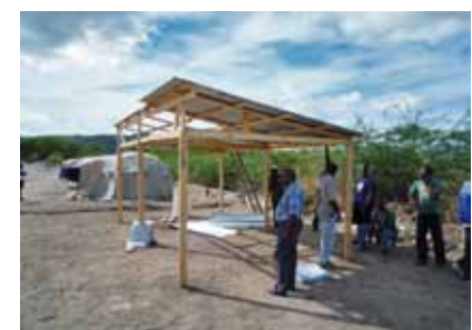
Prototype transitional shelter Photo: Joseph Ashmore
