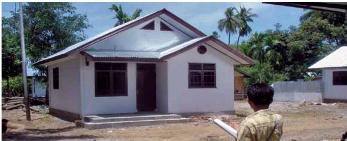
One of the completed shelters in Sigli, Aceh. Photo Joseph Ashmore
