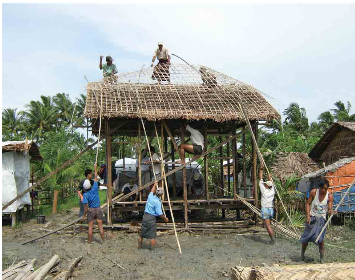
Covering bamboo canopy(Kyet-nin) over the roof ▲
