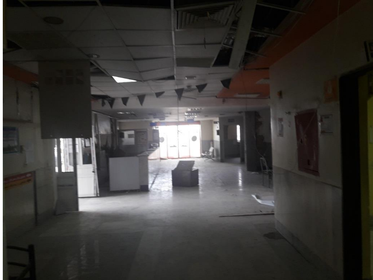
Failure of suspended ceilings, 2017 Kermanshah earthquake Sarpol'e Zahab Hospital (IIEES-2017).
