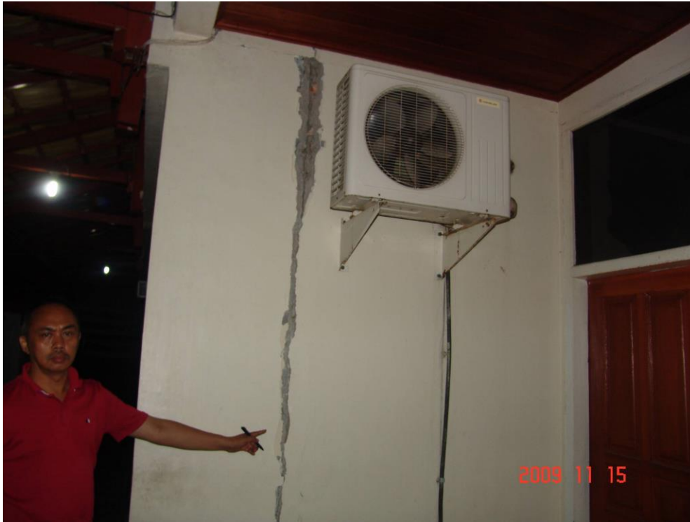
Crack at the contact point of RC column and infill wall, Ache, Indonesia (2009)
