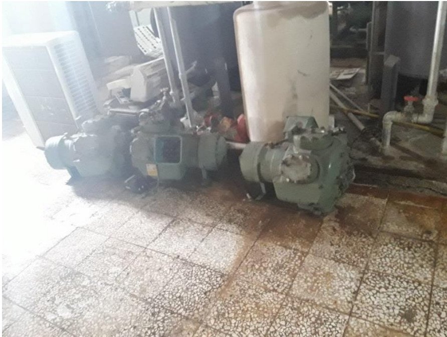
Damage to Water pumps, 2017 Kermanshah earthquake Ghasre Shirin Hospital (IIEES-2017).
