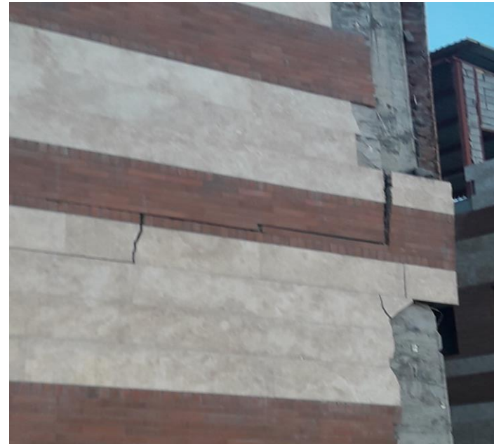
Adhered veneer damaged during 2017 Kermanshah earthquake Tazeh Abad Health Center, (IIEES-2017)
