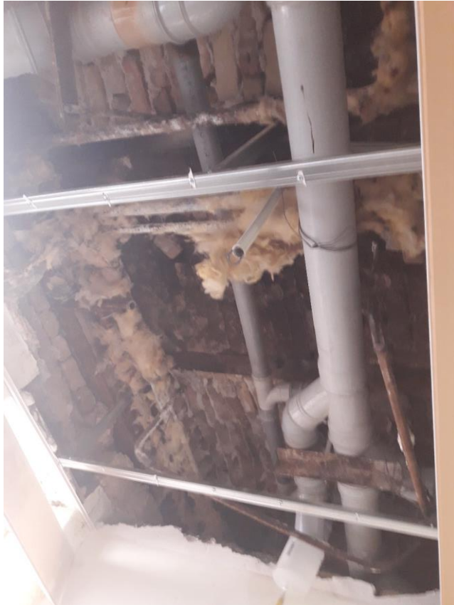
Swage breakage, 2017 Kermanshah earthquake Paveh Hospital (IIEES-2017).
