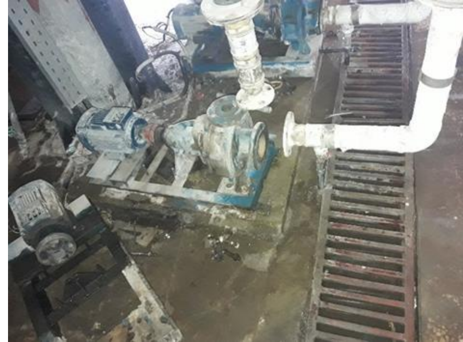
Damage to piping system, 2017 Kermanshah earthquake Ghasre Shirin Hospital (IIEES-2017).
