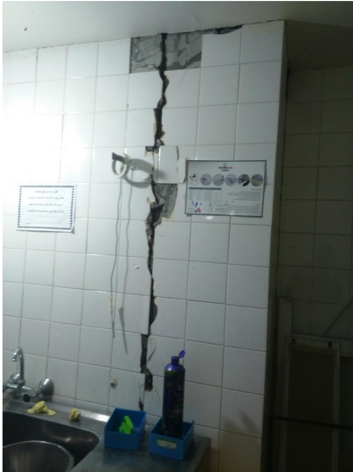
Damage to interior walls, 2017 Kermanshah earthquake Javanrood Hospital (IIEES- 2017).
