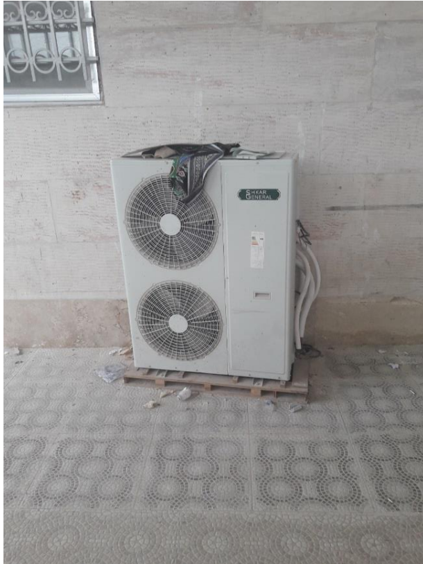
Damage HVAC Equipment, 2017 Kermanshah earthquake Sarpol'e Zahab Hospital (IIEES-2017).
