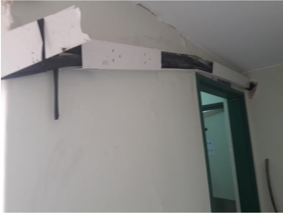
Damage to electricity channels, 2017 Kermanshah earthquake Ghasre Shirin Hospital (IIEES-2017)
