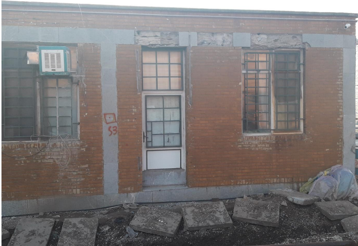
Adhered veneer damaged during 2017 Kermanshah earthquake Tazeh Abad Health Center, (IIEES-2017)
