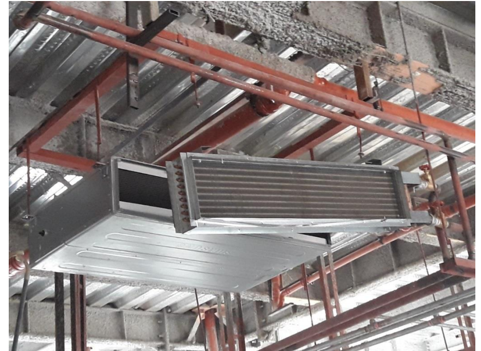
Damage to HVAC components, 2017 Kermanshah earthquake Sarpol'e Zahab Hospital (IIEES-2017).
