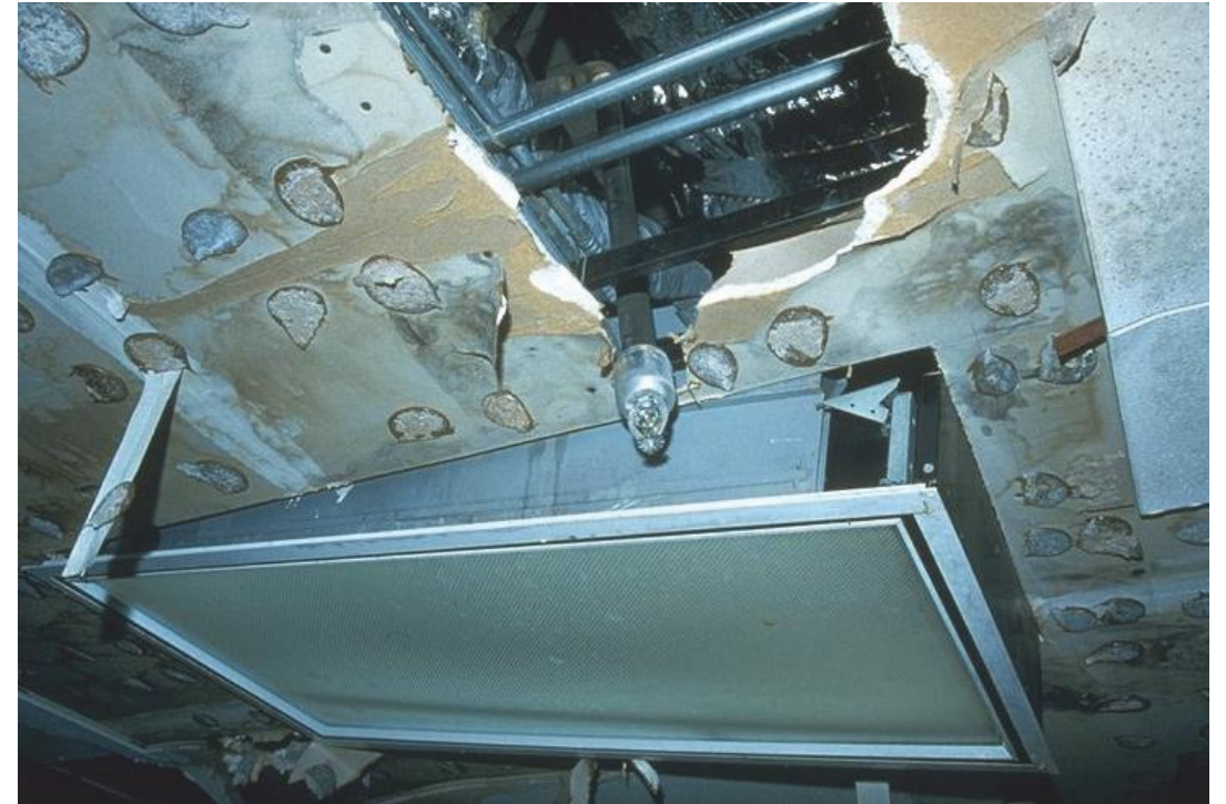
Fractured sprinkler line and dislodged light fixture in the Olive View Medical Center, 1994 Northridge earthquake (NISEE, 2016d).
