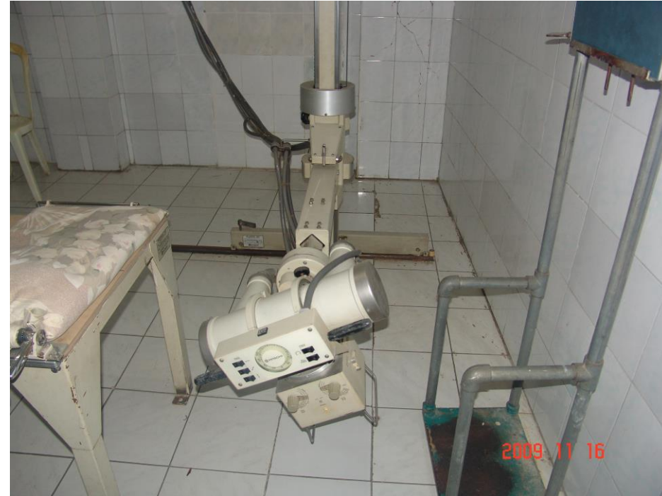
Damage to medical equipment, Selaguri hospital, Overturning and Damage to the X-ray equipment observed 2009 Ache earthquake (IIEES, 2009)
