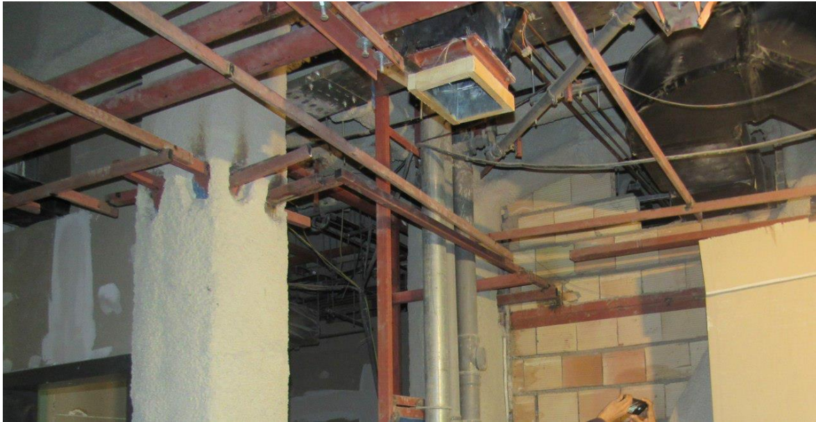
Figure 12. samples of architectural and mechanical elements in Non-Structural assessment
